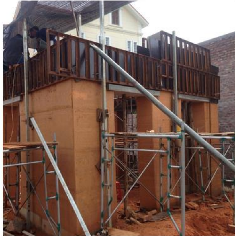
5. Installing lintel and joining formwork to connect wall base
