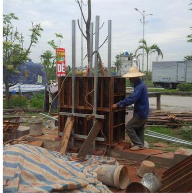
2. Put earth in to ready-made formwork (made of steel shape + board)
