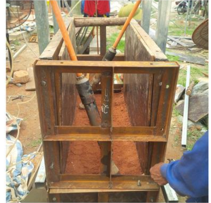
3. Compacting earth with small-sized and easy-to-use pneumatic rammer
