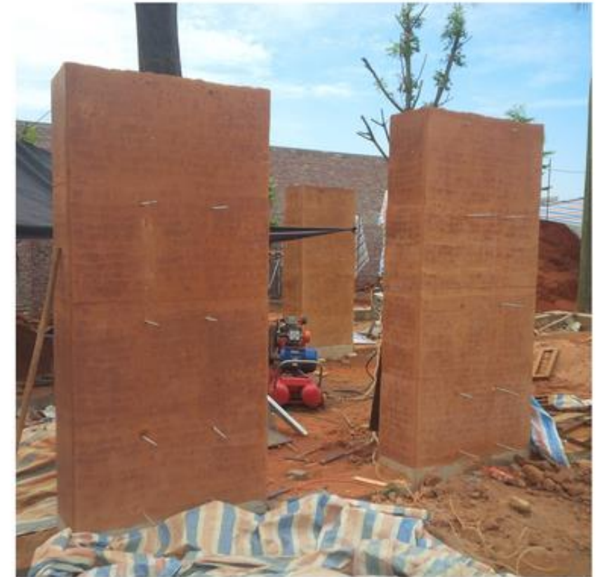
4. Lower wall after removing formwork
